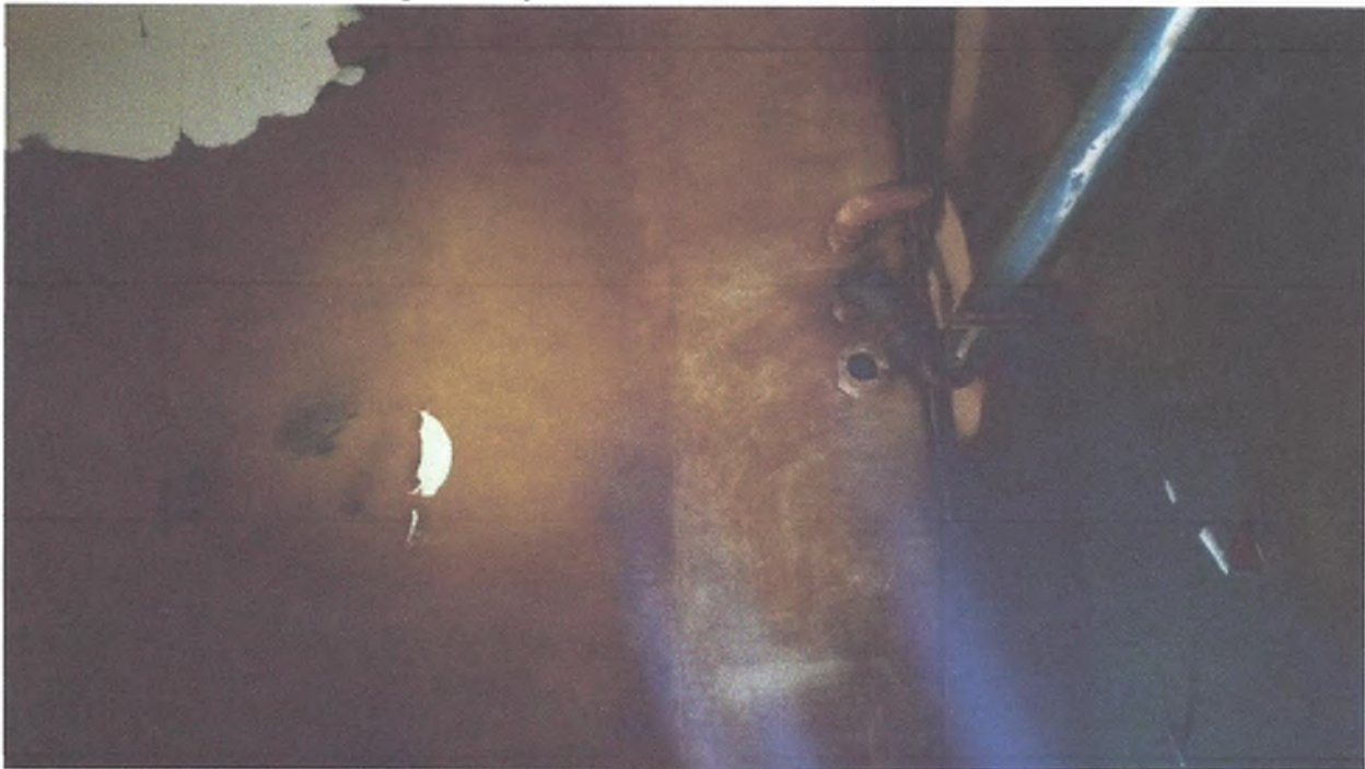
(9) Condition of Tank Upon Entry the second time.
