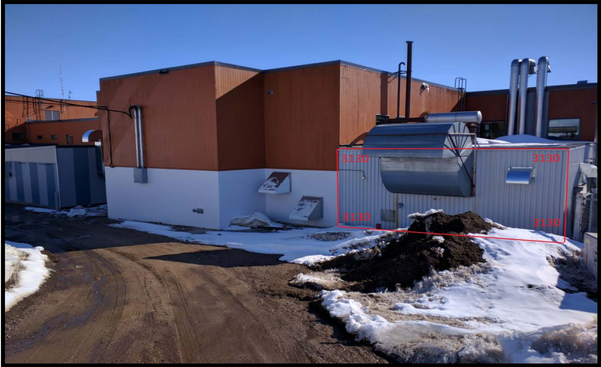
Figure 2: External view of Room 3130 / wall to be expanded.
